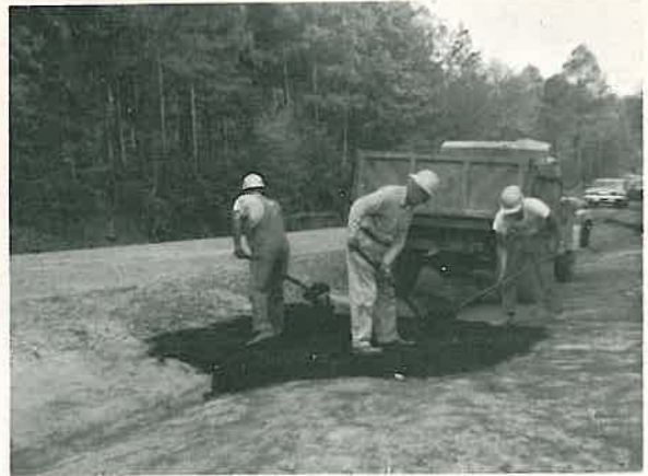
Spreading and shaping ditch check on State Highway 32, southeast of Hope.
