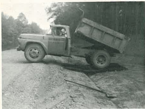
Compaction of ditch check
