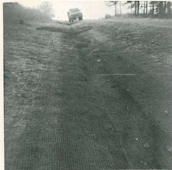
Jute matting placed between ditch check southeast of Hope.
